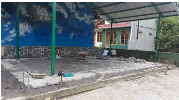
Gambar 13. Proses *pavingisasi*
