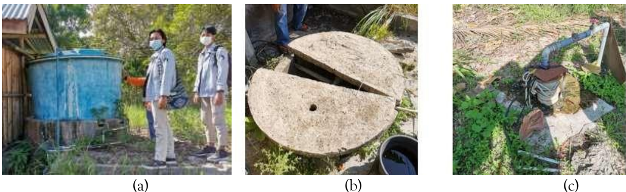
Gambar 3. Kondisi Jaringan SPAMDes (a) Bak Pelepas Tekan, (b) Sumur Gali, (c) Sumur Bor
